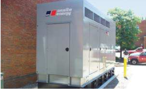
A newly installed MTU Onsite Energy 350 kW generator set features a Level 3 sound-attenuation enclosure.
